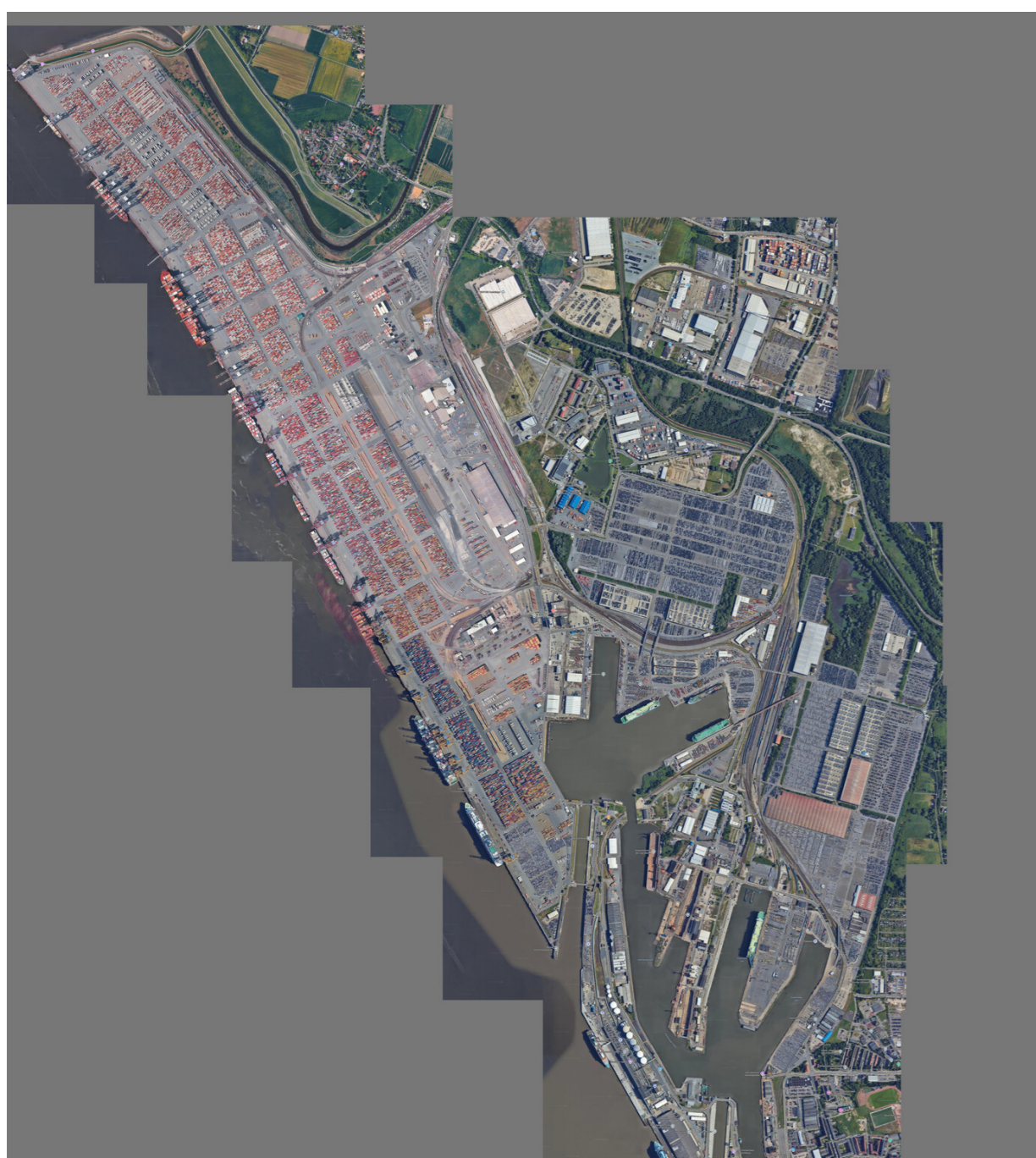
Figure 1: Satellite image of the Port of Bremerhaven showing the full extent of the port infrastructure [1].
